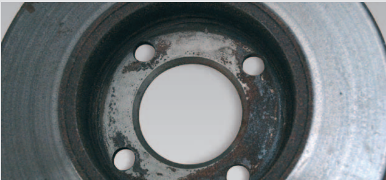
► Heavy underlying corrosion
